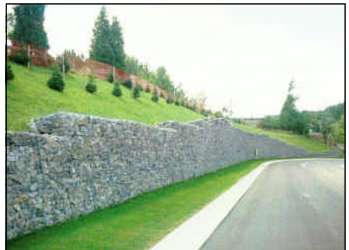
Example of gabion wall
