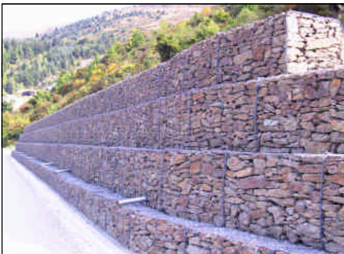
Example of gabion wall
