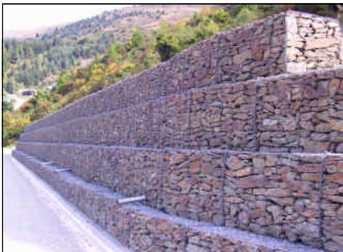
Example of gabion wall
