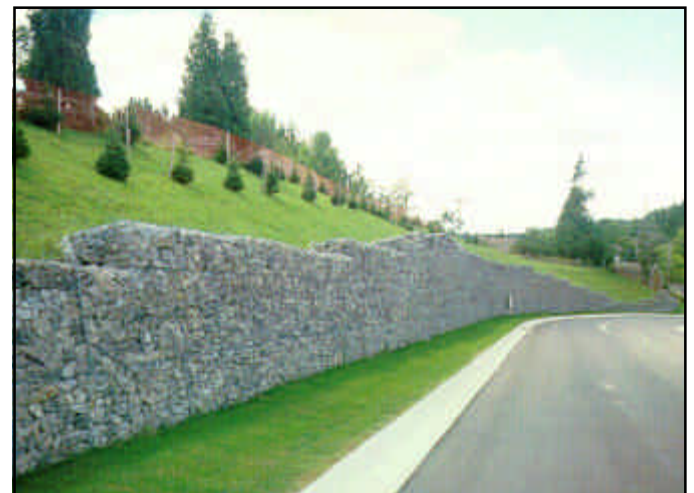
Example of gabion wall
